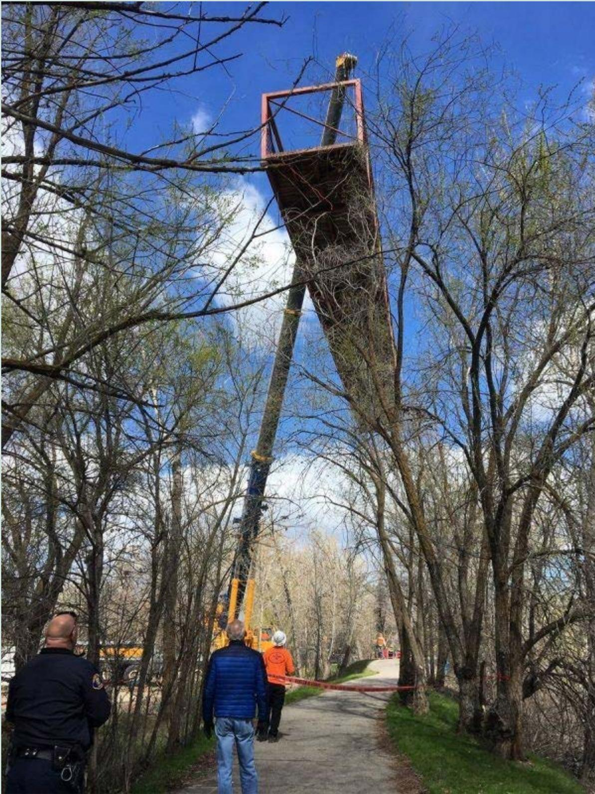
A crane hoists the Plantation Greenbelt bridge off of its footings in April 2017 for safety reasons during high-water flood flows that spring.
